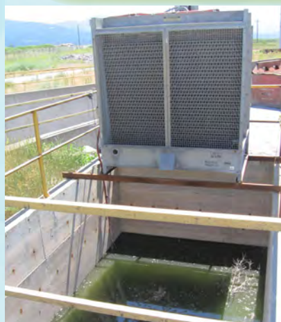
Passive wastewater evaporation pond
