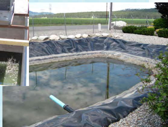
Passive wastewater evaporation pond
