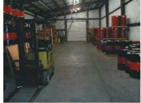
Figure 3 Concrete Floor Sloped to Center
