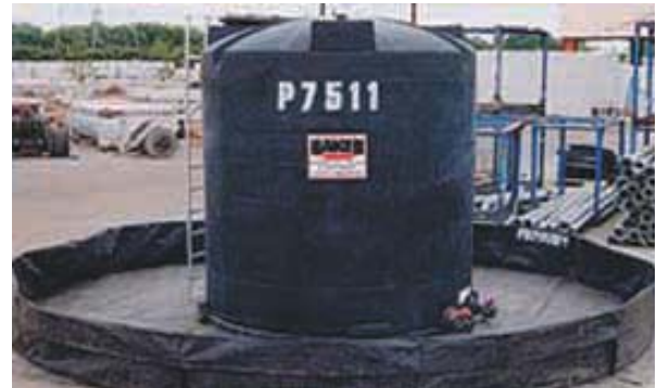
Figure 34 Synthetic secondary liner
