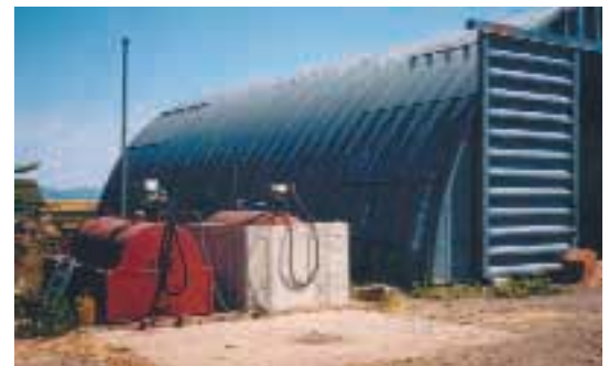
Figure 13 Small on/off loading pad with blind sump.
