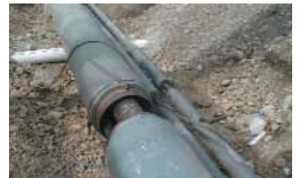
Figure 19 Example of double wall piping.
