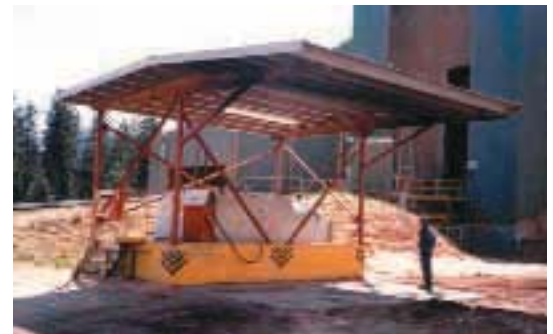
Figure 12 On/off loading pad with blind sumps.
