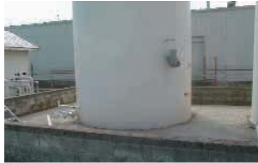
Figure 1 Concrete Block Secondary Containment
