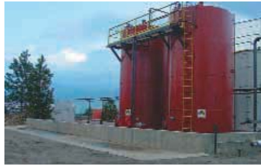
Figure 2 Solid Pour Concrete Secondary Containment
