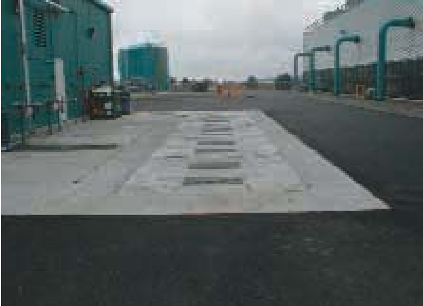
Figure 7 Loading platform that slopes to the center.
