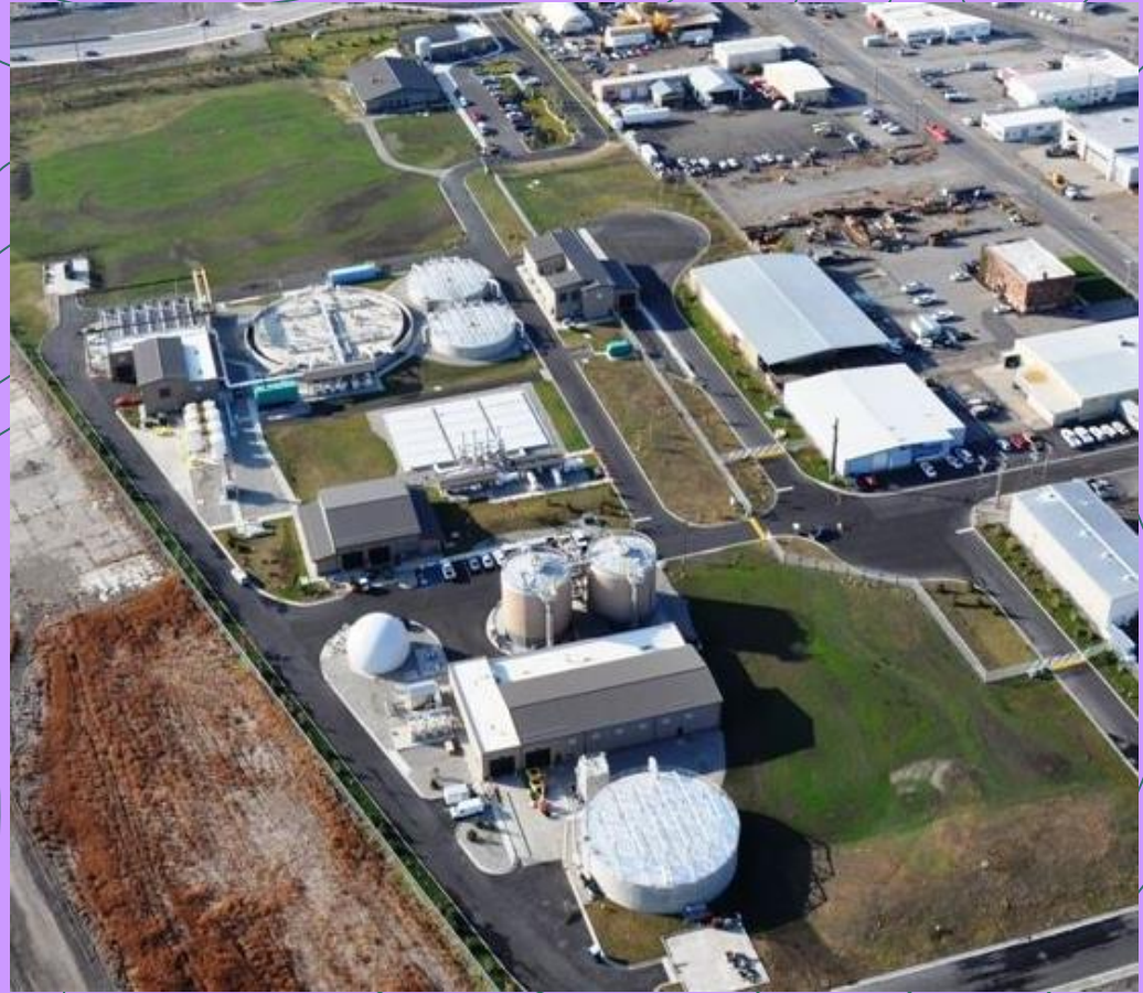
Spokane County Regional Water Reclamation Facility
